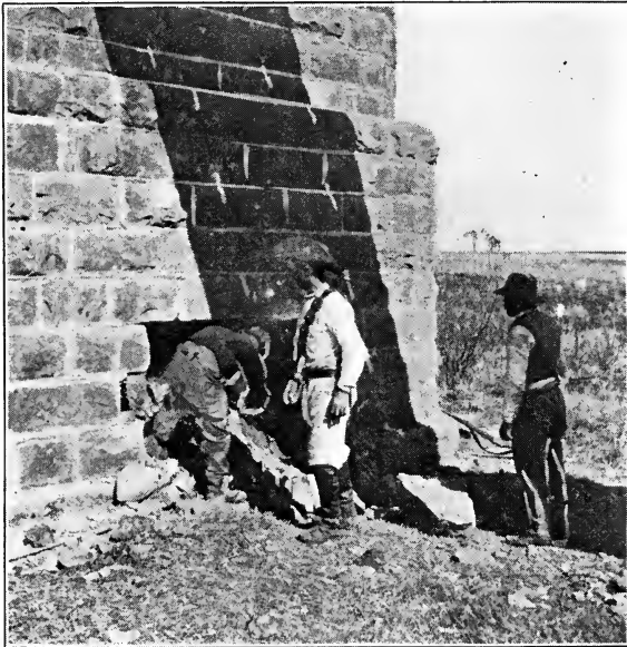
The Italian Dynamite Brigade mining the piers of the Oliphant River bridge.
